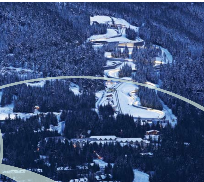
The Whistler Sliding Centre will be home to training, international competition and tourism.
