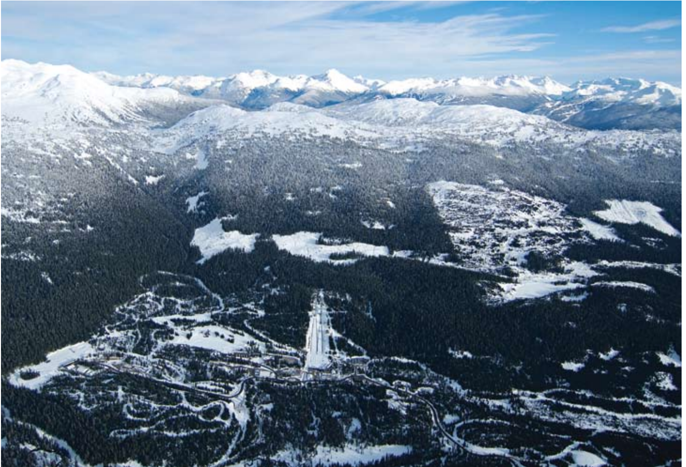
Whistler Olympic Park will provide recreational users and athletes of all levels and abilities with access to over 70km of cross country trails.
