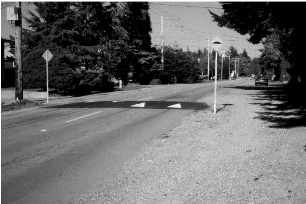
Figure 7.3 Speed Hump on Road Without Curbs
