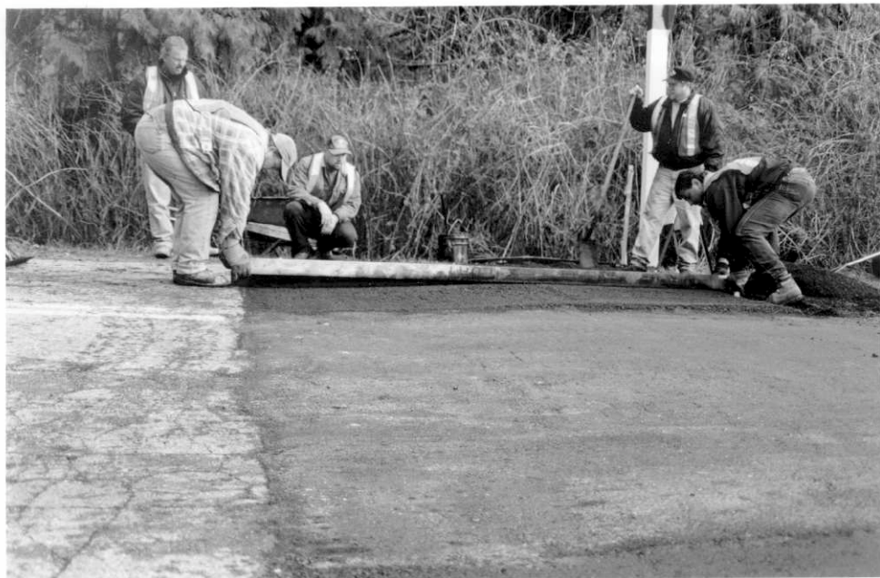
Figure 7.9 Shaping a Speed Hump With a Template
