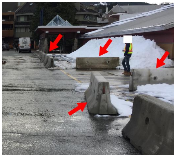
Photo #1 – Partial View of Concrete Barriers
