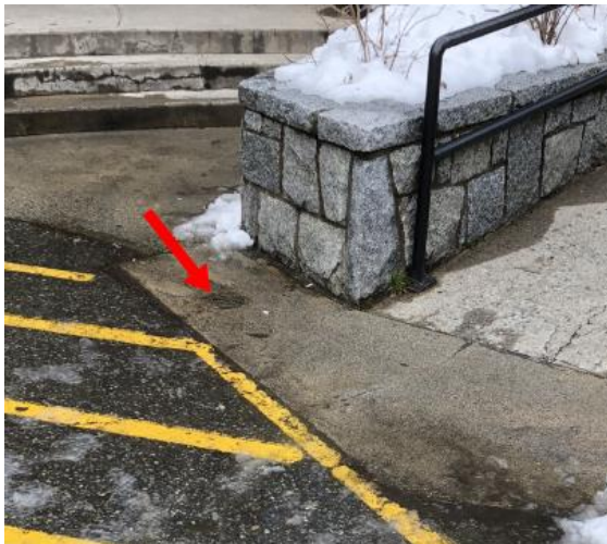
Photo #2 – Western Ramp Drain
