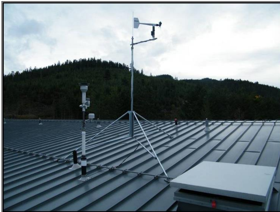
Figure 4 Tripod Mounted Anemometer and BAM Inlet located on the Roof of the HPC building
