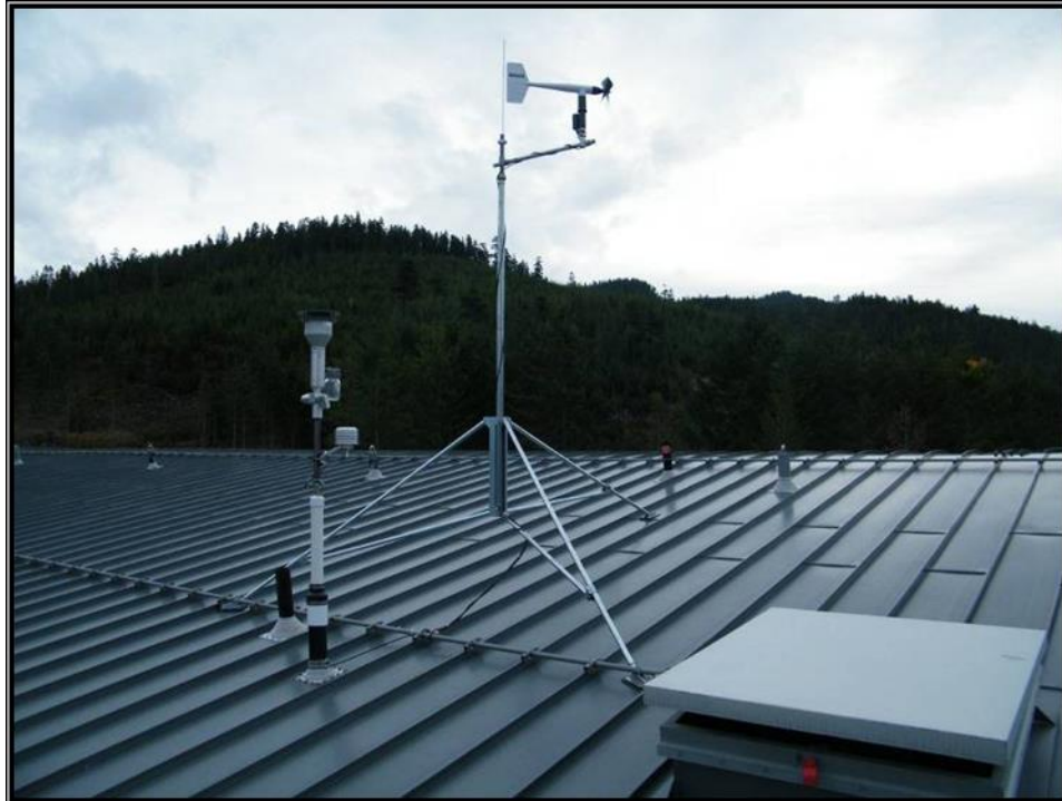
Figure 4 Tripod Mounted Anemometer and BAM Inlet located on the Roof of the HPC building
