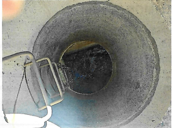
Photo 2: Manhole access to WWTP effluent outfall pipe, May 15, 2023.
