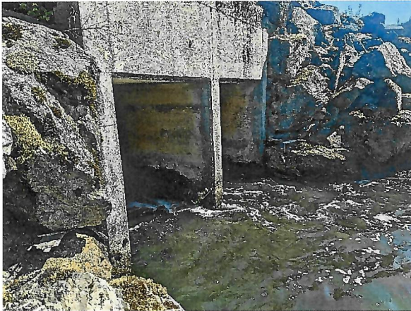
Photo 5: WWTP outfall interior, May 15, 2023.
