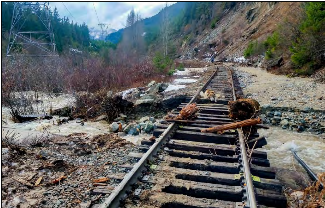
Photo 5-15. Flooding on November 23, 2017 washed out the railway tracks at Sproatt Creek.
