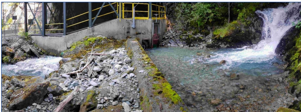
Photo 5-9. The water intake on Blackcomb Creek at 860 m. The natural streambed is interrupted by the dam (middle of the photo) and water flow is directed towards the intake (middle top). There is very little flow in the water at the uphill edge of the dam.
