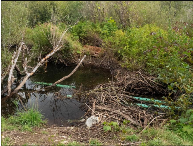
Photo 6-42. These perforated pipes lower water levels at this dam beside the new Valley Trail in the Miller Creek Wetlands.
