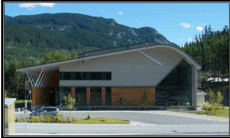
Figure 1 High Performance Centre (HPC) in Cheakamus Crossing Neighbourhood
