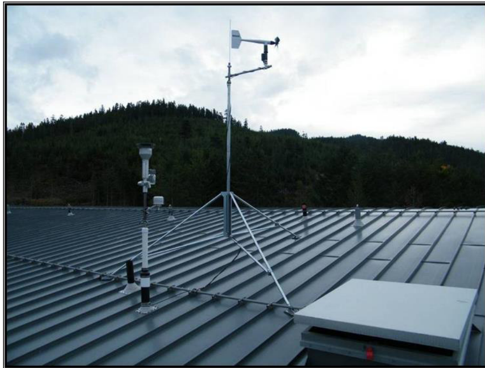
Figure 4 Tripod Mounted Anemometer and TEOM Inlet located on the Roof of the HPC building
