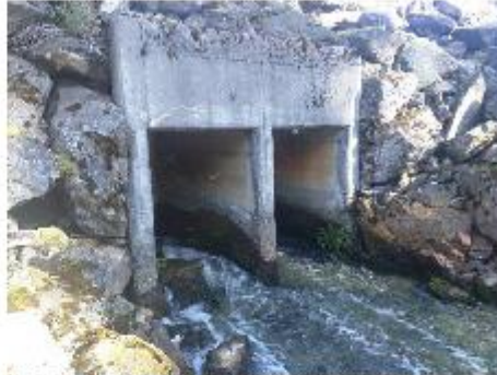
Photo 6: WWTP outfall interior, October 17, 2018.
