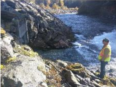
Photo 5: WWTP effluent outfall viewing downstream, October 17, 2018.
