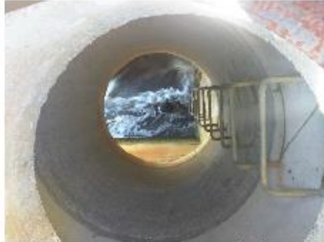
Photo 2: Manhole access to WWTP effluent outfall pipe, October 17, 2018.
