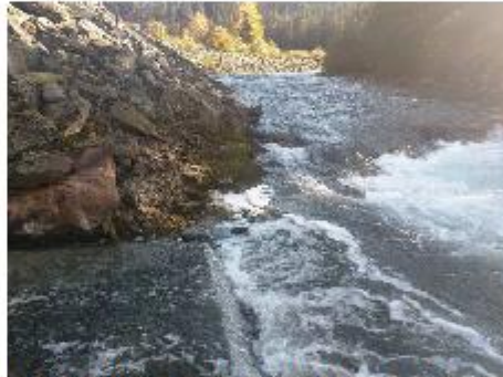
Photo 4: WWTP effluent location in Cheakamus River, showing upstream baffle, October 17, 2018.
