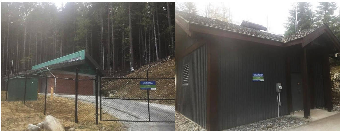
Figure 6: Left; 21 Mile Creek pumphouse and treatment station on Alta Lake Road with poor vegetation setbacks. Right: Taluswood pumphouse roofed in cedar shakes.
