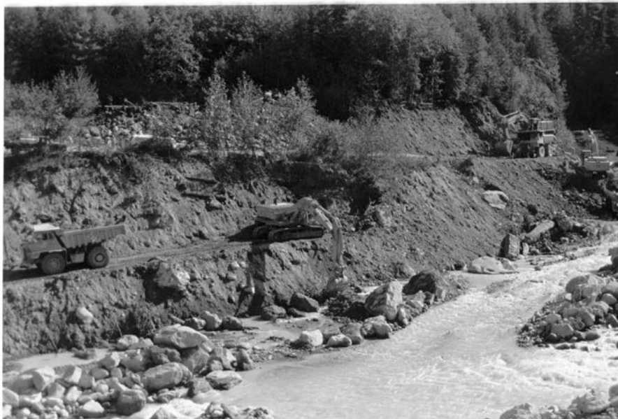
Photo Credit to Whistler Question from Whistler Museum Rechannelization work and extensive rip-rapping upstream from the Culliton Creek Bridge began September 23, 1991. The $450,000 repair job became necessary when flood waters forced closure of the span, 40 km south of Whistler.
