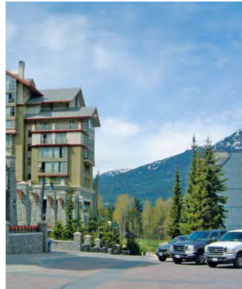
Springs Lane drop-off, looking east to golf course and Westin Plaza
