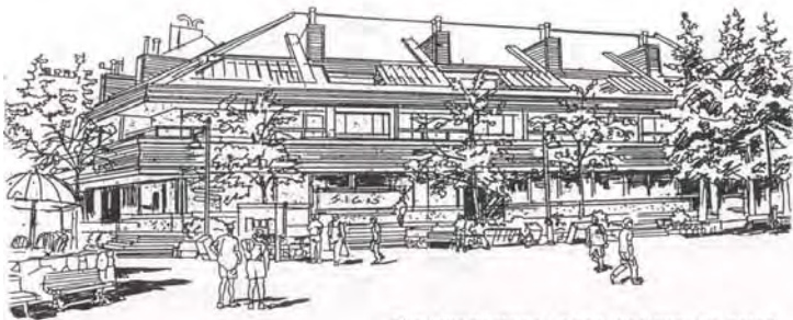
The Hearthstone Lodge, designed by noted Canadian architect Arthur Erickson, is an example of a "Heritage" building.
