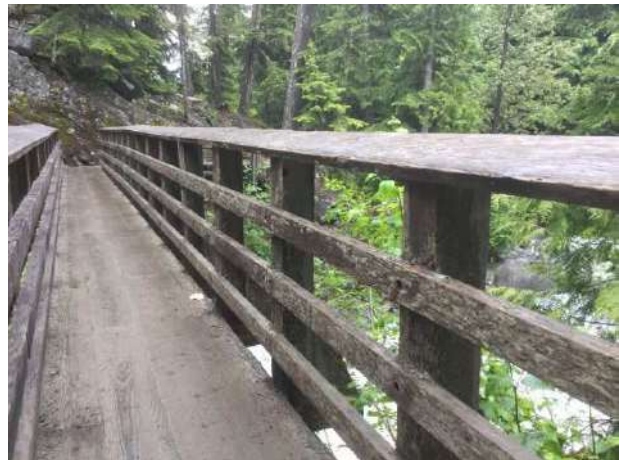
Photo 6 Typical handrail condition
