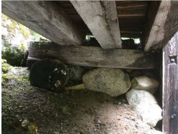
Photo 13 North approach boardwalk
