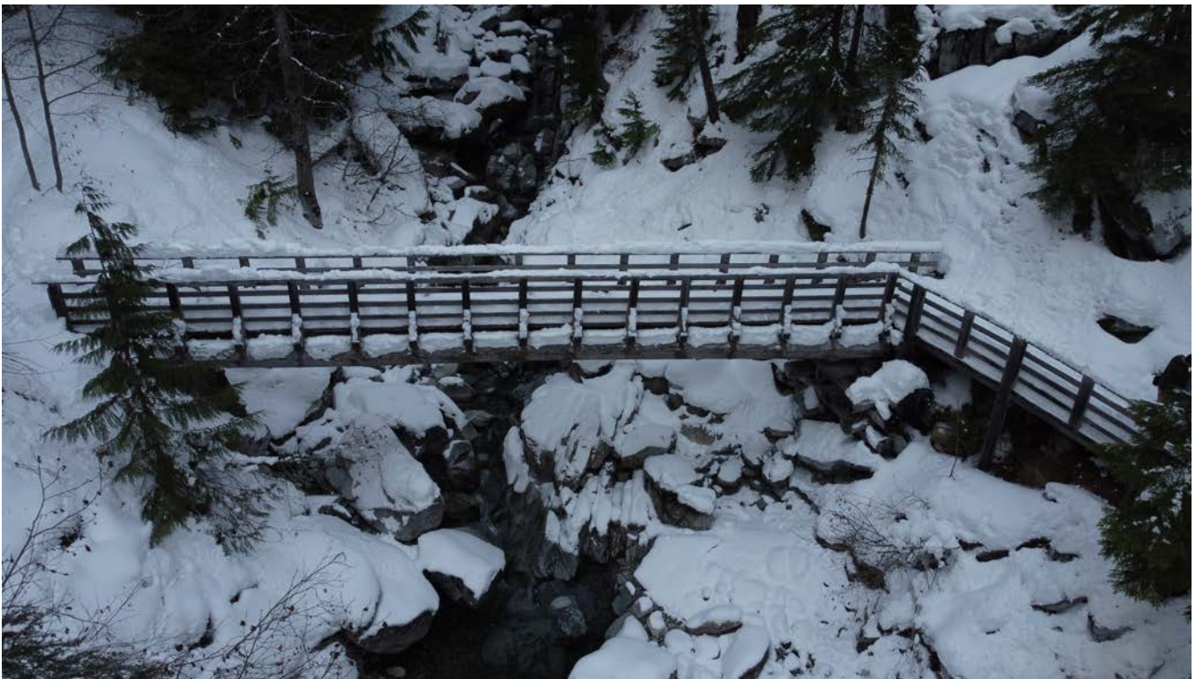
Photo 2: Overview of study area looking upstream at existing Flank Trail bridge
