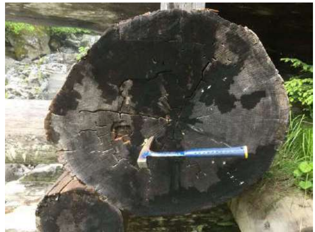
Photo 10 North abutment sill
