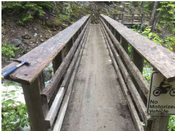
Photo 5 Typical deck condition
