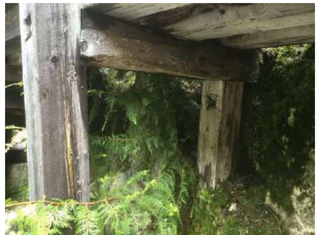
Photo 12 North approach boardwalk
