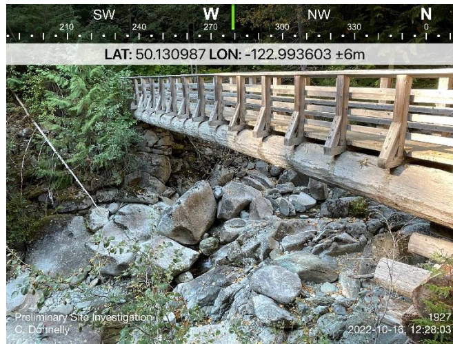
Figure 1: Southwest creek bank. Existing bridge is supported on stacked rocks on top of bedrock or large boulders.
