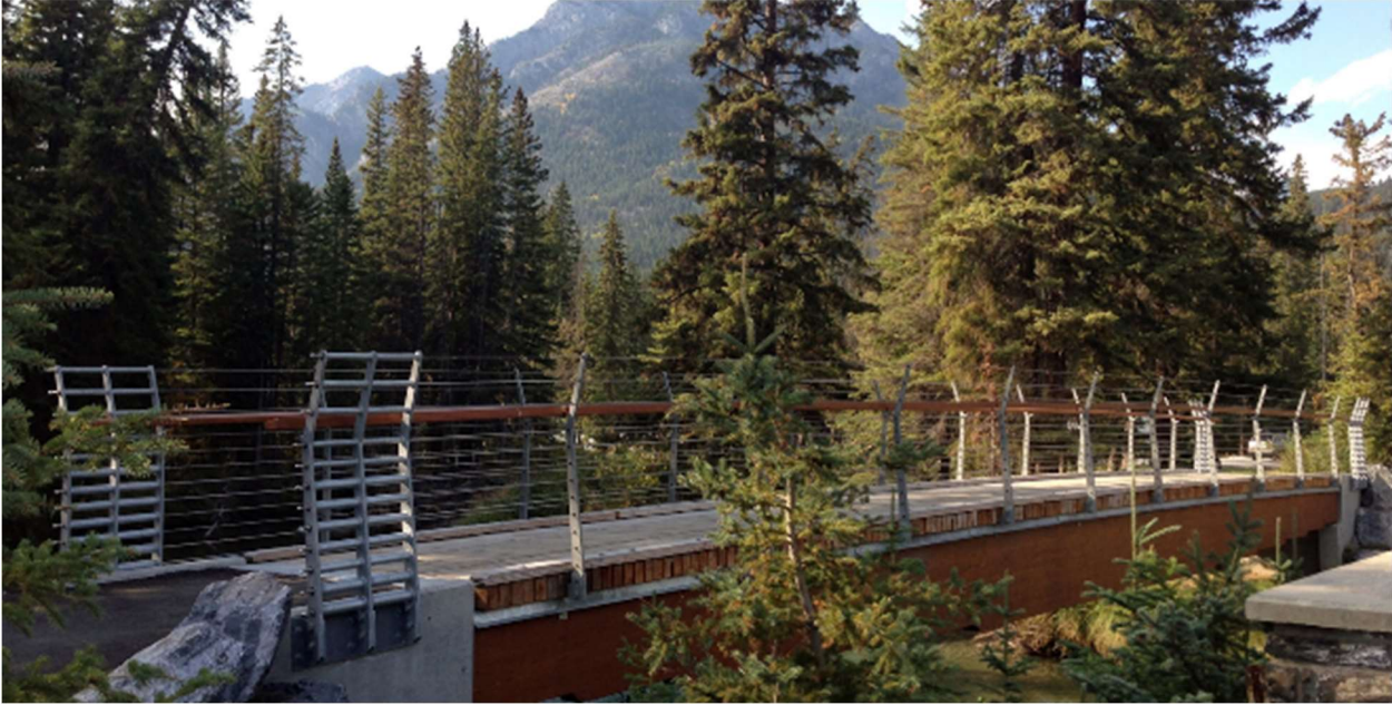
Legacy Trail Glulam Bridge, Banff Ab.
