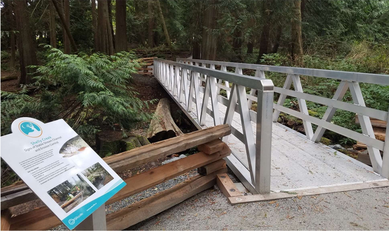
Shelly Creek, Aluminum Truss Bridge, Parksville BC
