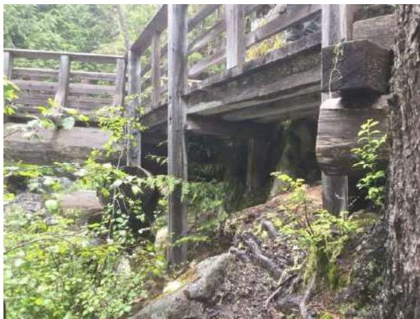
Photo 11 North approach boardwalk
