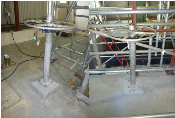
Main Gate valves and actuators (Inlet valves)
