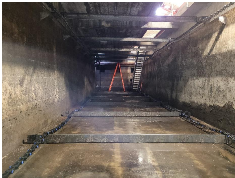
Figure 3: Concrete Tank, PST1
