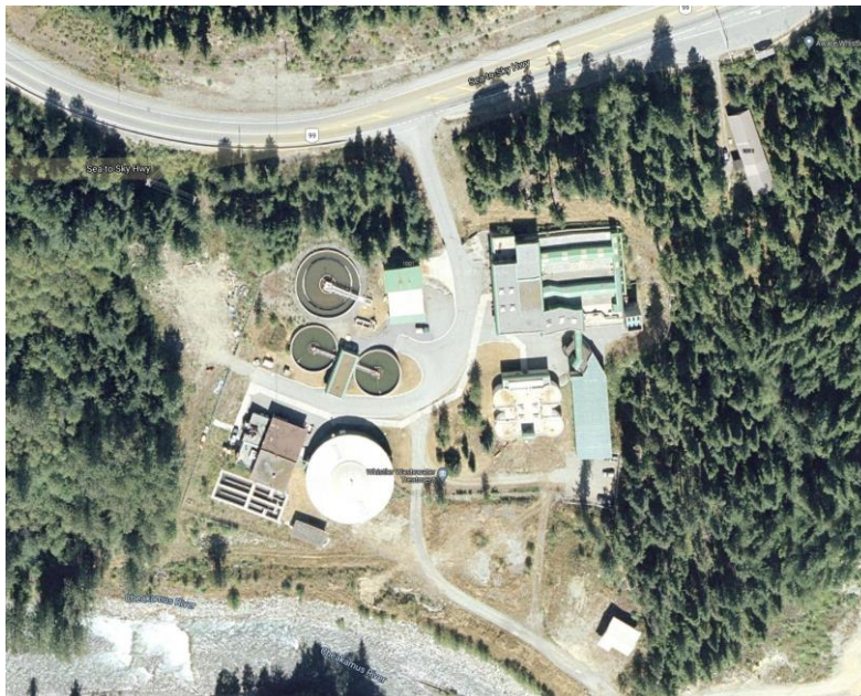
Figure 1: Location of RMOw Waste Water Treatment Plant (Courtesy of Google Maps)
