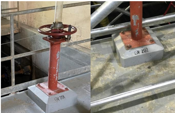
Main Gate valves and actuators (Inlet valves)
