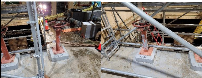
Main Gate valves and actuators (Inlet valves)
