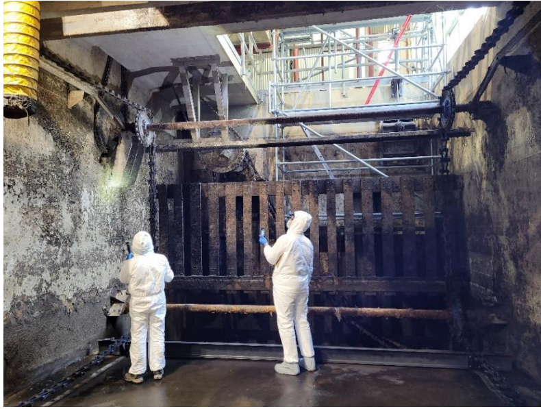
Figure 2: Inspection in PST1
