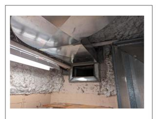
Removal of all old ductwork + duct insulation, pipework, and vent grills where possible
