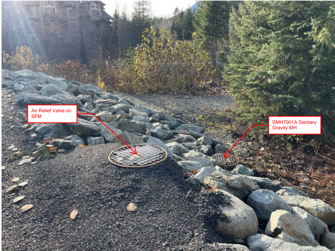
Photo S2-10.1: Clusters S2-10a, S2-10b & S2-11 General Location Looking Towards Fitzsimmons Creek from Dike Berm.
