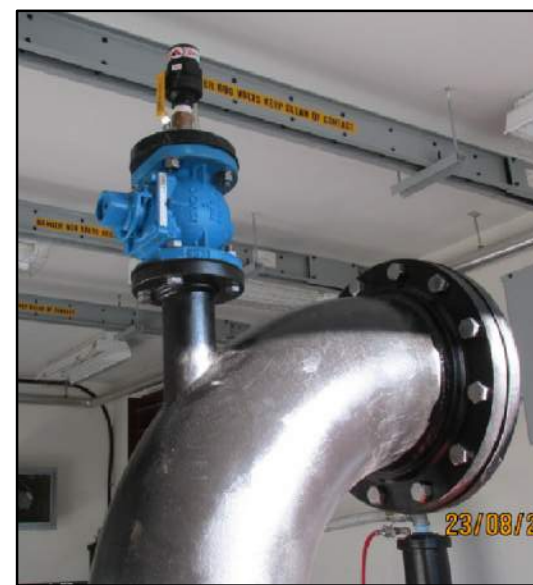
AIR VALVE ON PIGGING PORT LAUNCH ELBOW
