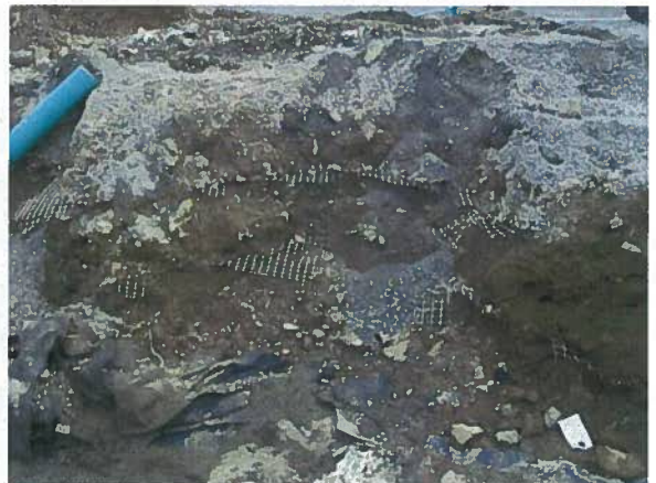
Photograph 4: Overburden Materials above Geomembrane (May 10, 2011)
