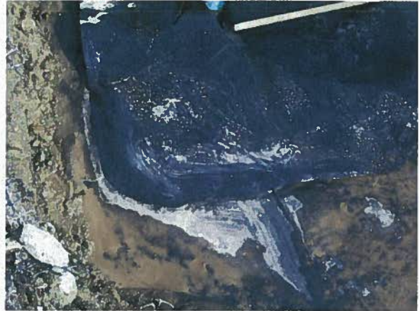
Photograph 8: Extrusion Welding of Seam (May 13, 2011)
