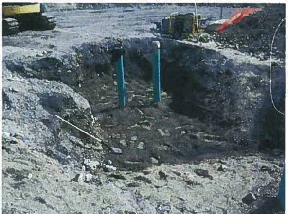
Photograph 12: Soil Backfill in Excavation (May 18, 2011)
