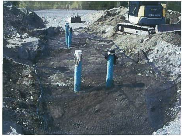
Photograph 14 Placement of Geogrid in Excavation (May 18, 2011)
