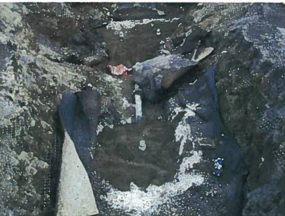
Photograph 3: Valves Backfilled with Bentonite Powder and Soil (May 9, 2011)
