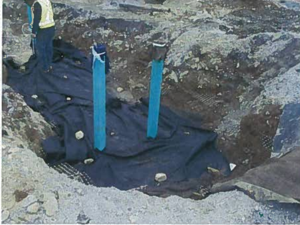
Photograph 7: Excavation Covered with Geotextile (May 10, 2011)
