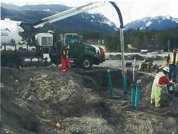
Photograph 11: Vacuum Truck Used to Clean Geomembrane (May 18, 2011)
