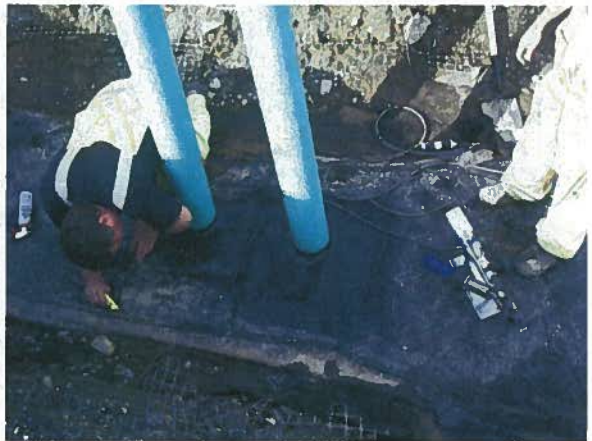
Photograph 10: Boots over PVC Pipe Penetrations (May 13, 2011)
