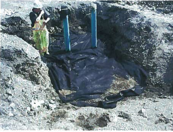
Photograph 13 Placement of Geotextile in Excavation (May 18, 2011)
