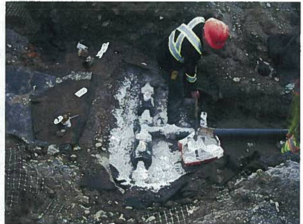
Photograph 2: Sealing of Valves and "Tee" Connection with Bentonite Powder (May 9, 2011)
