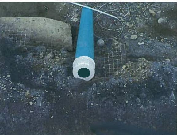
Photograph 5: 150 mm Diameter PVC Pipe and End Cap (May 10, 2011)
