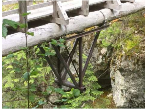
Photo 11 Undertruss
