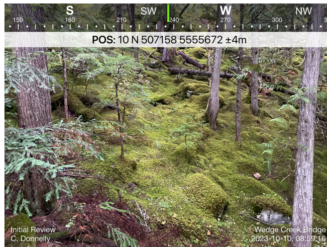
Figure 3: Slope located approximately 18 m behind the southwest bridge abutment.
