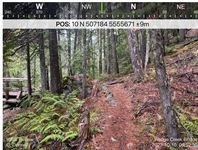
Figure 6: Slope behind the northeast bridge abutment.
