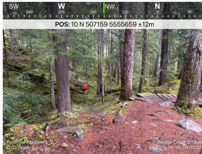
Figure 1: Southwest side of the existing bridge – shallow depression to the west of the woodwork leading to the bridge.
