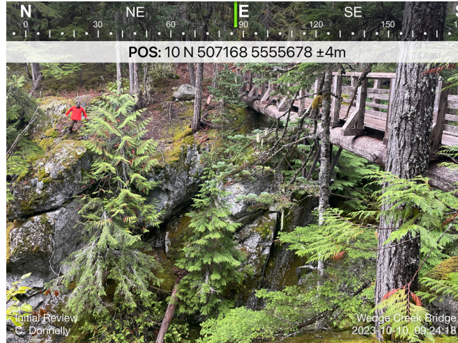
Figure 5: Exposed bedrock beneath the northeast bridge abutment.
