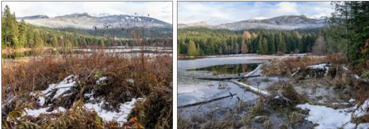
Photo 2- 29. (left) Lost Lake Lodge 1 at the north end of the lake; (right) Lost Lake Lodge 3 is nearer the main beach at the outlet to Blackcomb Creek. While structurally sound, it has not been occupied since 2020.
