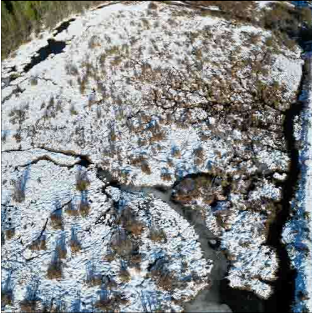
Photo 2-11. Aerial view facing north of RW5 channel (foreground) and RW6 channel (top left). The ditch (right side) parallels the adjacent rail line, and is impounded by three large dams.
